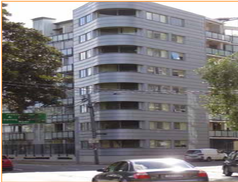
City West Housing project Pyrmont NSW
